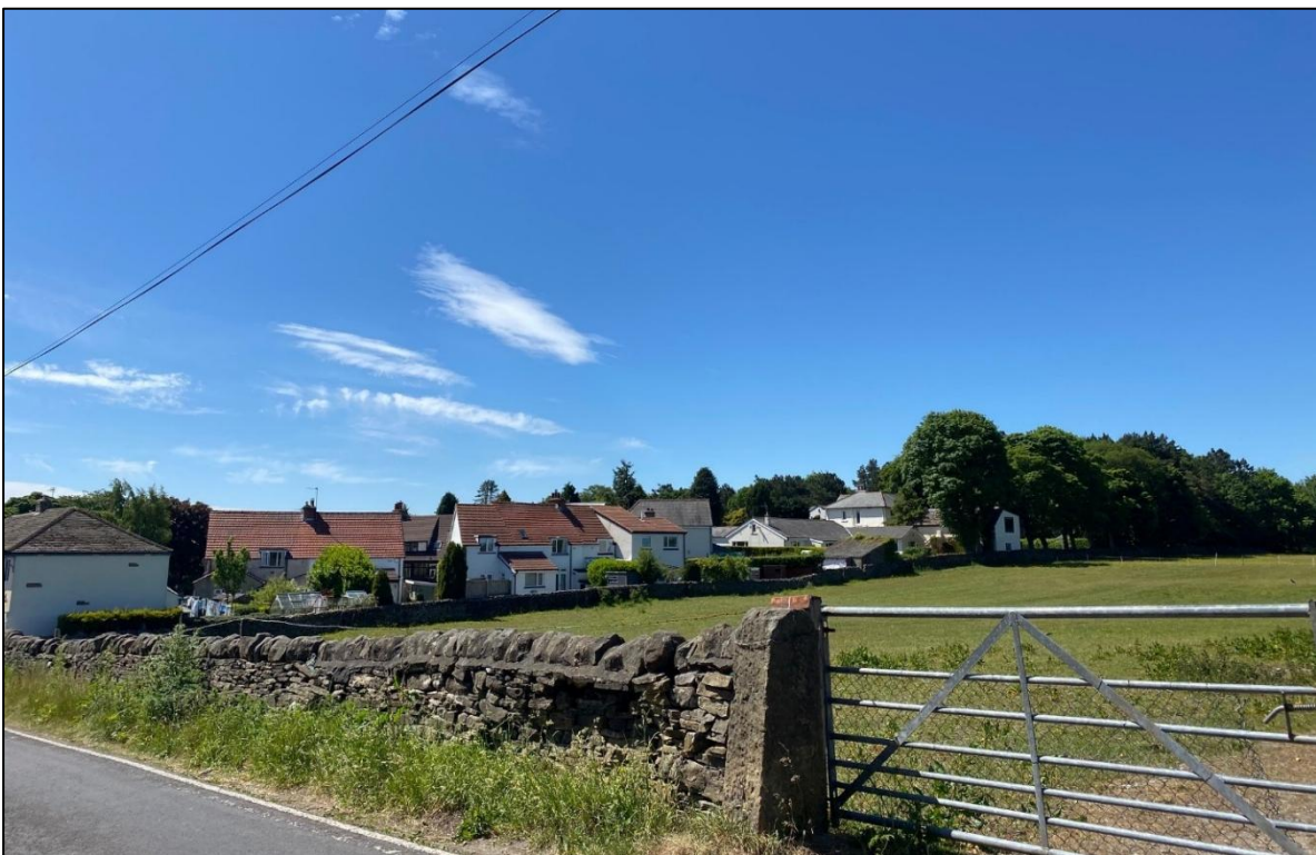
Figure 2 BA/013 Looking South West
